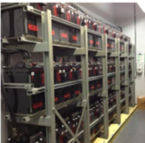
Figure 3 - 3-tier open rack with top terminal cells and seismic bracing.
