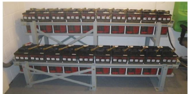
Figure 2 - 2-step open rack with top terminal cells
