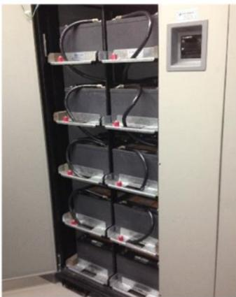
Figure 1 - Battery cabinet with top terminal cells
